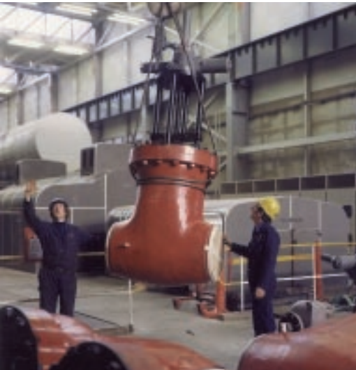
A 30" Class 300 DEWRANCE Parallel Slide Valve being installed in a UK Power Station.
