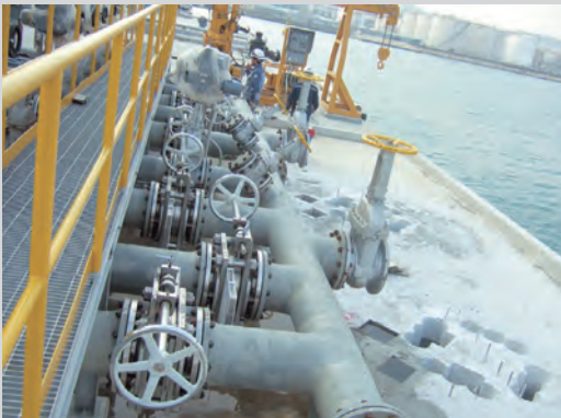
■ A loading arm construction (S-Oil in Korea)
