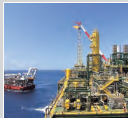
• Flooding Production Storage and Offloading •
